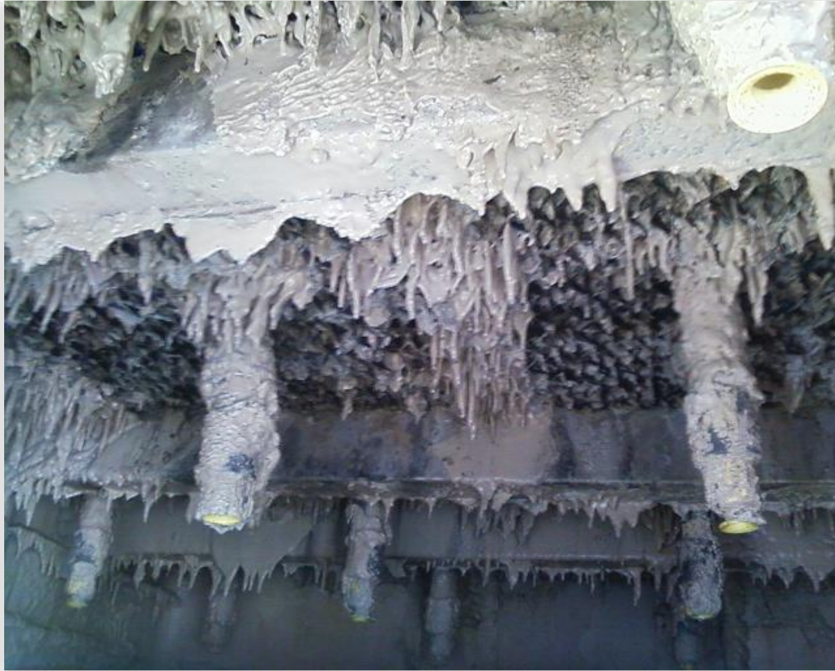
Splash grids clogged with paper fibres at a pulp and paper mill
